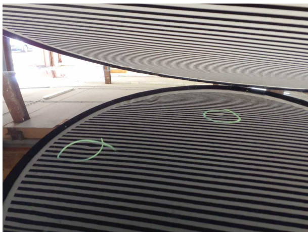
Damage #4: Roof: Roof - dent(s) - Smooth repair work
