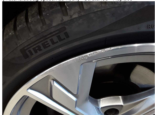
Damage #13: Wheel / tyres: Alloy rim - front left side (Materialabtrag optisch zu hoch) - Scratched - Replace
