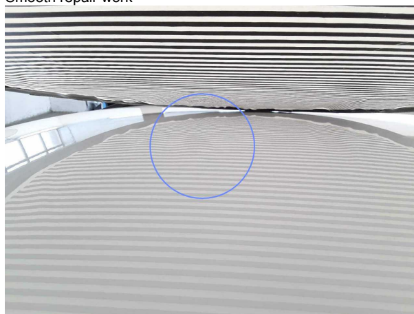
Damage #3: Roof: Roof - dent(s) - Smooth repair work
