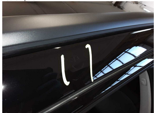
Damage #3: Roof: Roof rail - right side - Paint defect - Repair and paint
